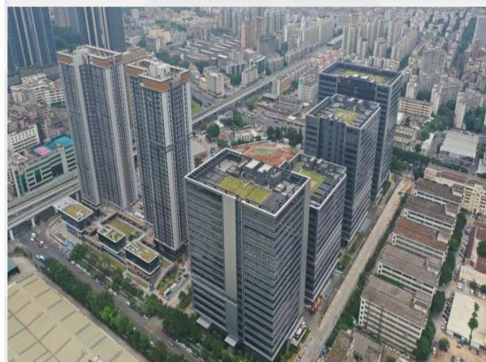
深圳建泰城市更新項目最新實景(2026) KS urban-renewal, latest site view (2026)
